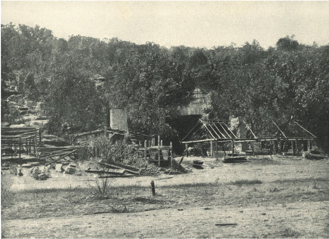
Nickajack Cave, southeast of Pelham, on the edge of Nickajack Lake, was one of the largest Confederate nitrate mining operations in the area. This September 1863 image depicts the cave entrance and some of the abandoned works after Confederates were forced from the area with the arrival of Federals in August. (photo from Vol. 4, The Photographic History of the Civil War , 1912, Francis Trevelyan Miller, editor)
